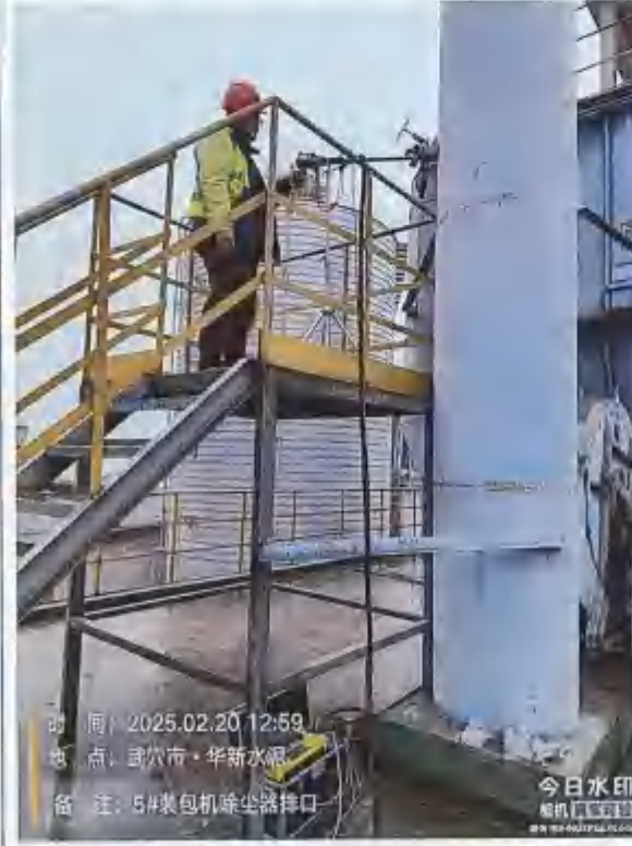
DA104-5#包装机除尘器废气排气筒
